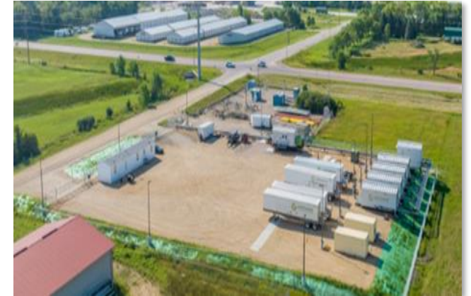
Permanent RNG Injection Station – Fixed pressure reduction and pipeline injection compressors injecting agricultural RNG into pipeline via Certarus injection facility
